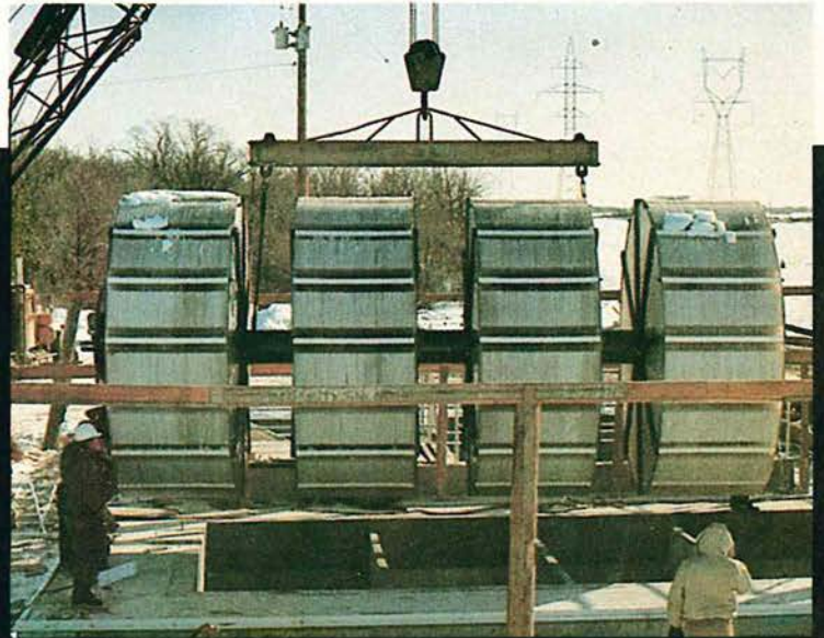
A rotating biological contactor sewage treatment unit at Norway House.
