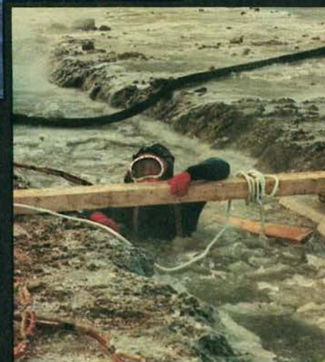
Laying 6" polyethelene water pipe across the Saskatchewan River at Nipawin. (Inset) Diver checking final installation.
