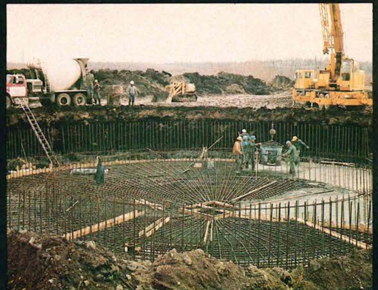
A rotating biological contactor sewage treatment unit at Norway House.
