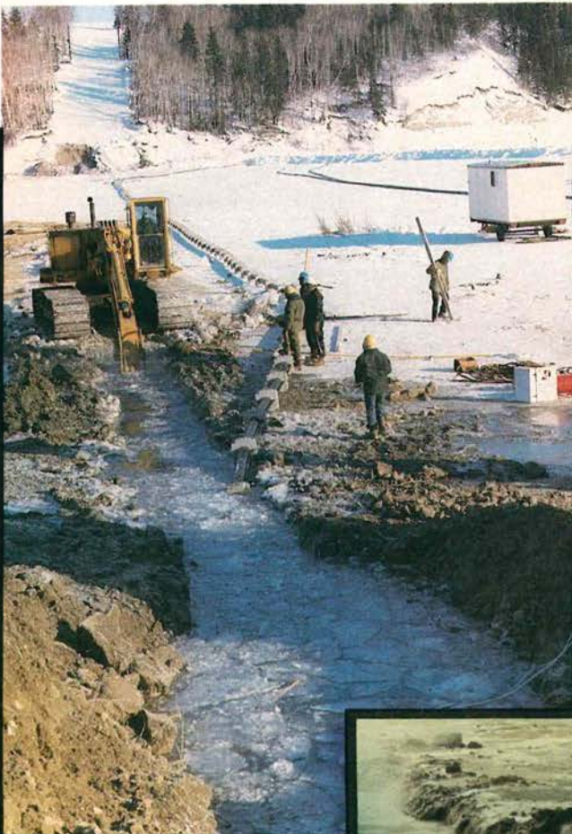
Laying 6" polyethelene water pipe across the Saskatchewan River at Nipawin. (Inset) Diver checking final installation.
